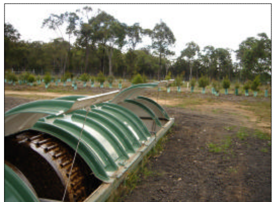
The Kelair-Blivet Model BL4000+2B during installation above. Below, the installed unit at Waratah Highlands Village, Bargo.
