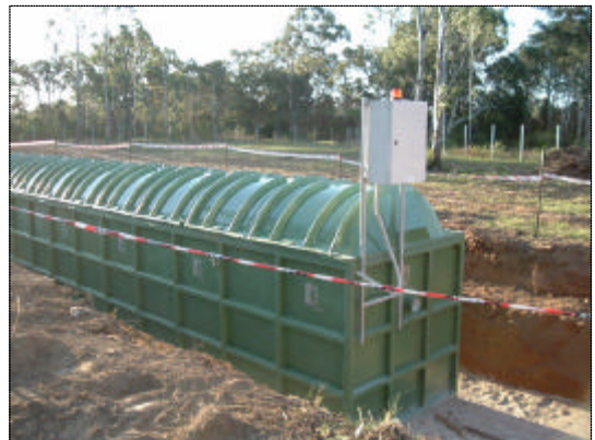
The Kelair-Blivet Model BL4000+2B during installation above. Below, the installed unit at Waratah Highlands Village, Bargo.
